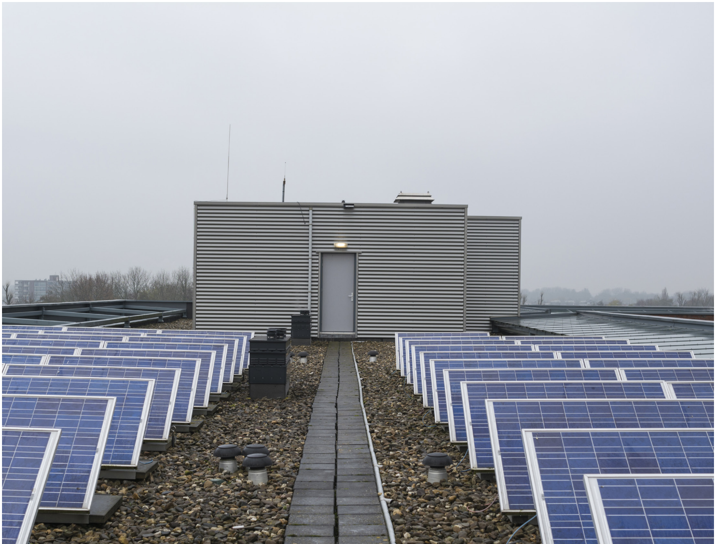
Solar panels connected to a battery storage system.
